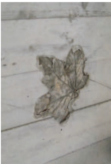
A wall built using self-compacting concrete showing grain of timber shuttering and the impression of a leaf placed in the formwork at the City & County Museum, Lincoln.
