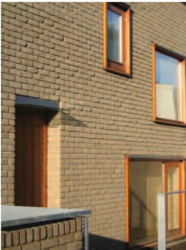
Whole brick reveal at front door and internal window linings expressing the thickness of the wall of house at Newington Green, London.
